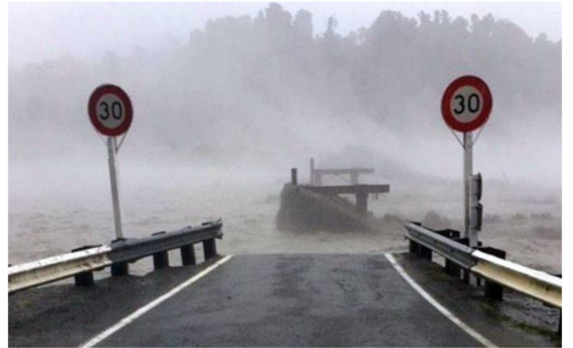
Figure 1: Waiho Bridge, Westcoast New Zealand, May 2019. © New Zealand Civil Defence West Coast
